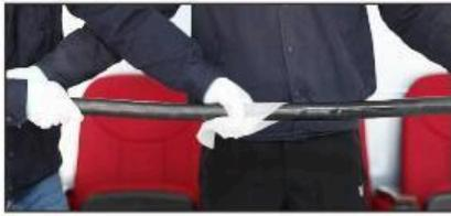
Clean the surface of cable, cable joints or other places to be protected;
