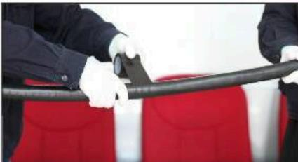
There is no front side or back side for the tape. It need to be spread out smoothly when wrapped, and do not fold or overlap;
