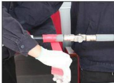
No lapping or wrinkle is allowed. Smooth out the tape when wrapping;
