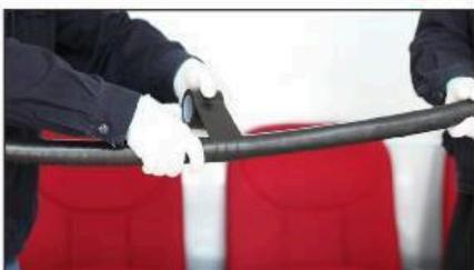
There is no front side or back side for the tape. It need to be spread out smoothly when wrapped, and do not fold or overlap;
