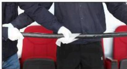
Clean the surface of cable, cable joints or other places to be protected;
