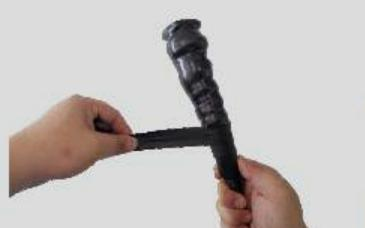
At the end of wrapping, pull and wrap the tape gently and press the tape end hard;
