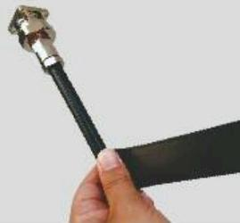
Keep the sticky side of tape towards the contact surface, stretching the tape to 3/4 of its width, and then spirally wrap it with a 50% overlap;
